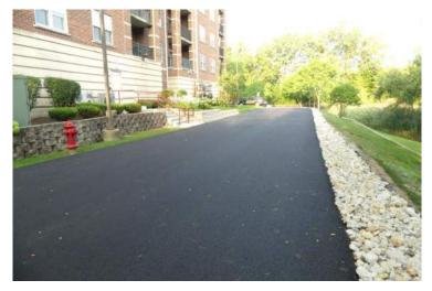
The Groves of Palatine Condominiums include four 7-story buildings constructed between 2002 and 2005. Road access to the rear of the northernmost building was only via an asphalt-paved fire lane, which had eroded due to the steep slope of adjacent grade.
